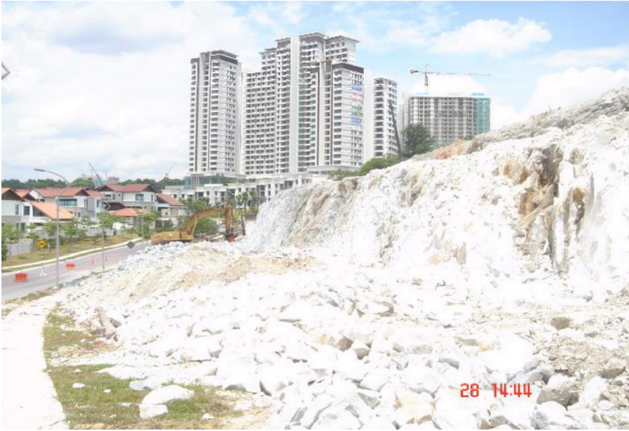
Hard materials were hacked by a hacking machine (b).
