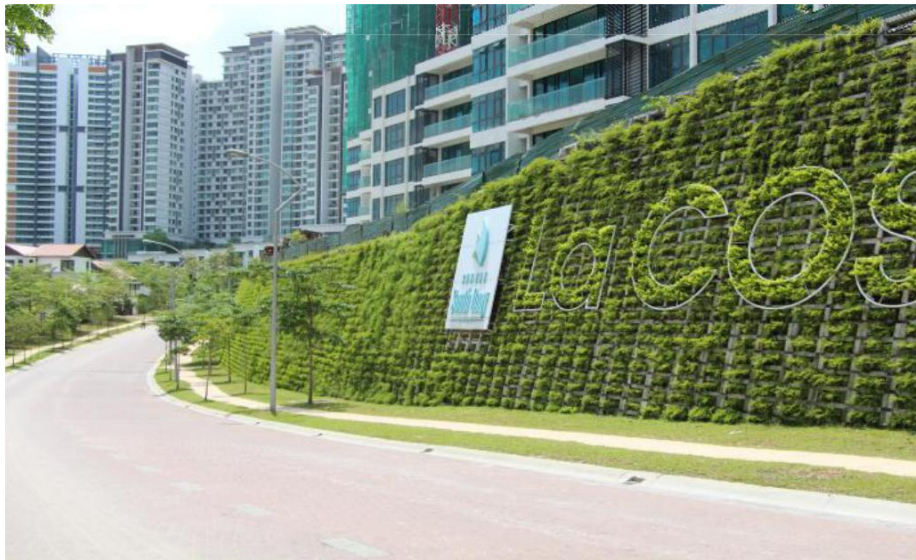
After Vegetation: Cribwall with creepers plant.
